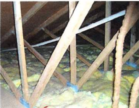
Loft insulation at 100mm
