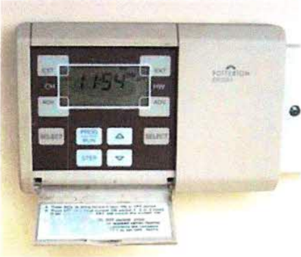
Boiler Controls
